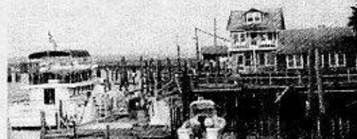
Second and third floors added in 1947. Second floor for storage and net repair. Third floor for truckers waiting to load shrimp.
