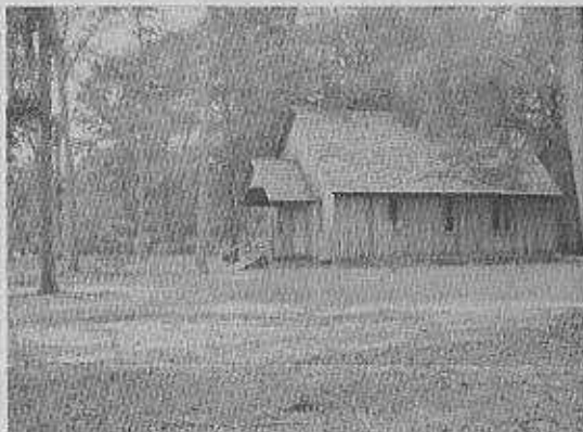
BURNT FORT CHAPEL WITH CEMETERY IN BACKGROUND.
